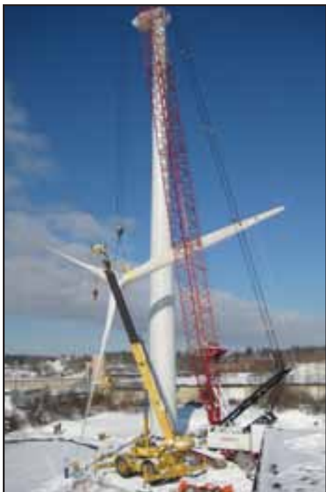
Hub and rotor erection
